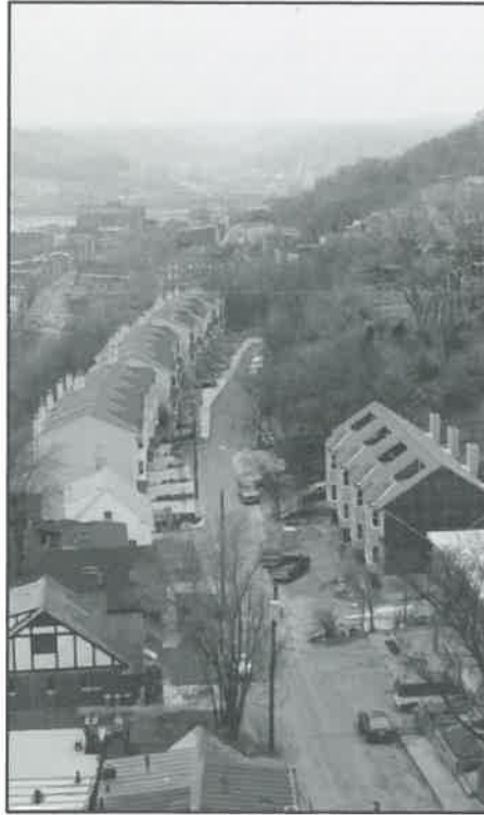
New housing construction on Uptown hillside
