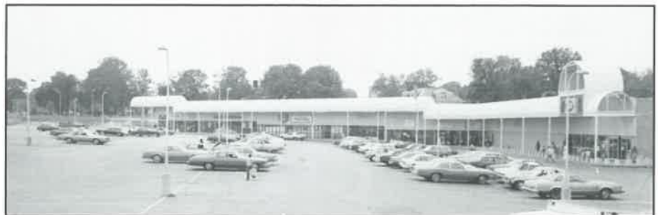
Avondale Town Center and Reading Road is the focus of Avondale's business district
