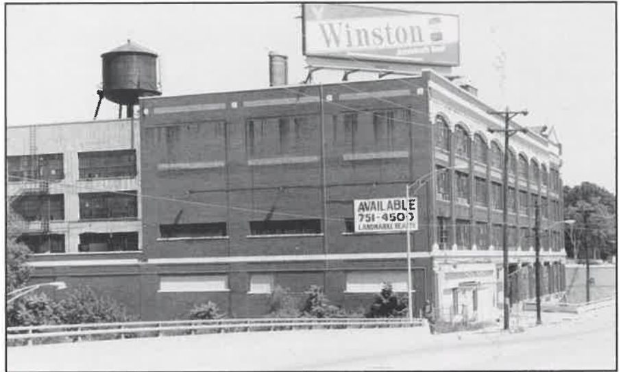
This former Ford Plant offers development opportunities, as do vacant nearby sites along the east side of I-71
