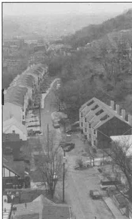
New housing construction
