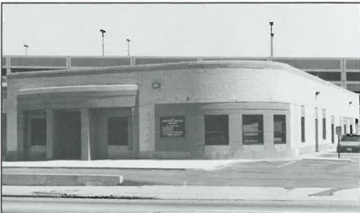
Some existing buildings can be adapted to new uses. (Former auto services center, now office uses.)
