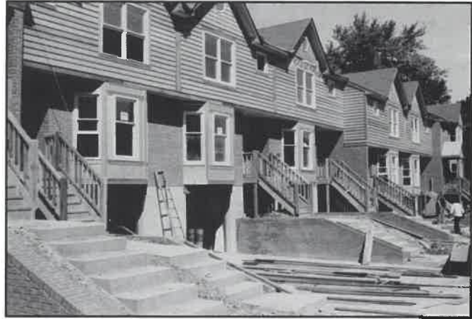
Rehabilitation and new construction provides jobs.
