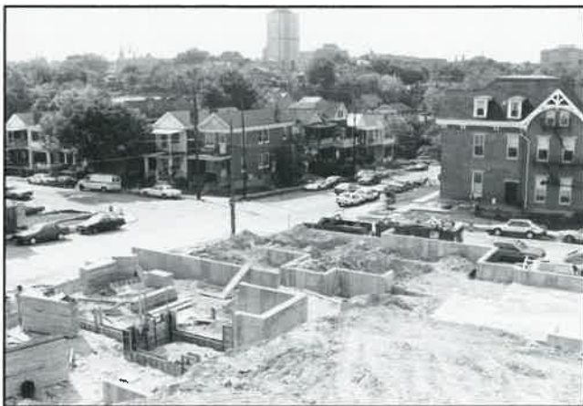
New housing construction in Corryville
