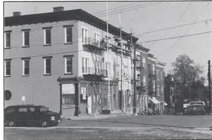
Housing rehabilitation in Mt. Auburn
