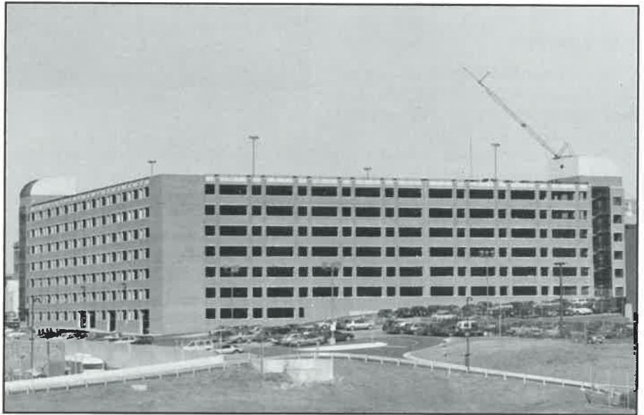
Garage under construction at the U.C. Medical campus (now completed)
